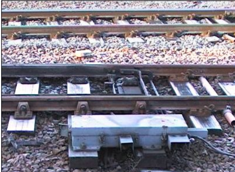
A point machine located adjacent to the switch blades it operates. Most point machines are electrically operated but London Underground has a large number of air operated machines.
